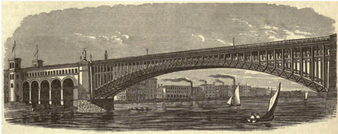
Figure 1: St. Louis Bridge
